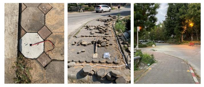
(Above left 06, center 07 and right 08) In order to install the flashing devices, the study attained permission from the university board to remove a series of paving stones approaching the field test site, and then a series of conduits were laid into the sand under the paving that houses the wiring system. Furthermore, a customed redesigned hexagon paving slabs was made that can house the electrical unit under each slab.
