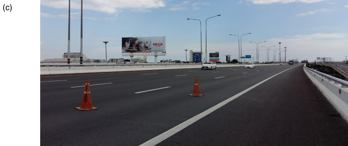
Fig. 1 Photo of Construction of the pilot test section: (a) key plan for the section and field test positions, (b) construction of the PA and (c) overview of the current porous pavement (photo taken in December 2022).
